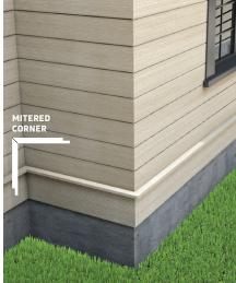
J Corner: Siding slides under corner Keep 1/16" gap between corner and siding No gap needed for vertical application
