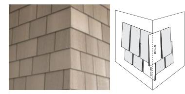
**Additional Fastening:** When shingles are going to be installed adjacent to and/or next to heat reflective surfaces, such as roofs, decks, solar reflective windows, metal flashings or blacktops, additional fastening is required. Sun and heat may cause shingles to lift or curl.
